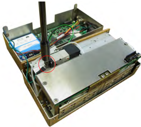
FIGURE 6.15: REMOVE THE GROUND WIRE
